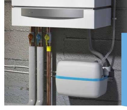
**SANICONDENS® Pro** pumps condensate away from condensing boilers and air conditioners. Small, this powerful pumping unit can be floor or wall mounted.
